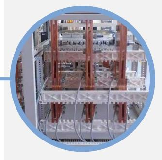
To meet the exacting specifications, Bensons manufactured the ACB section as a stand-alone item. This meant it could be installed in one corner of the plantroom next to the dividing wall leading to the engine section. This also positioned the ACB adjacently to the outside wall for the transformer cables.
